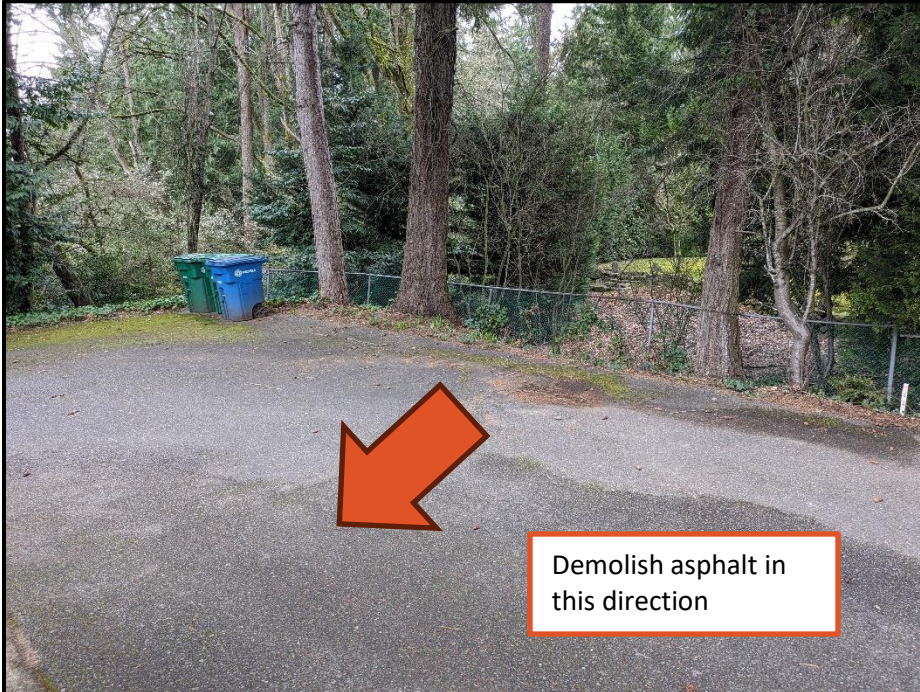
Photo 4. Base of tree 38 viewed from the south. The driveway is proposed for removal in this area. I recommend the asphalt removal begins closest to the tree and moves backwards. Once the pavement is removed no machinery traffic or materials are allowed. I recommend the project arborist is called if any large roots over 2-inches diameter are encountered.
